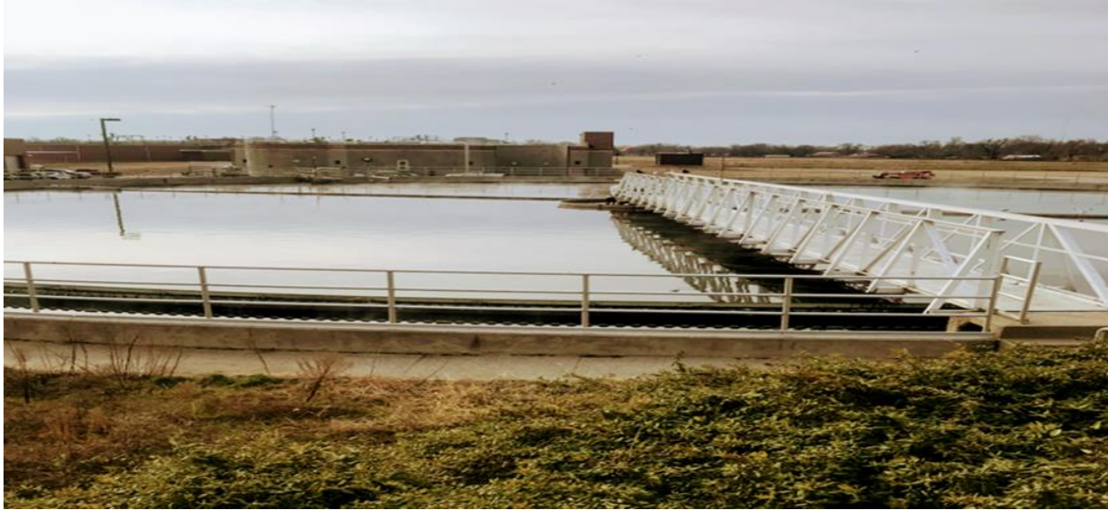
Figure 2.5. Wichita Wastewater Treatment Facility in 2018
