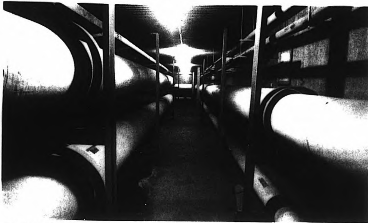
Heating and cooling pipes that service the Life Science Building are in a tunnel starting below the power plant. (Photo by Brian Corn)
